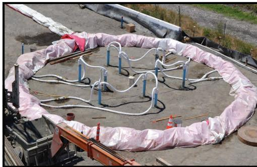
Close-up of freezing pipes going 128ft into the ground forming the retrieval shaft.
