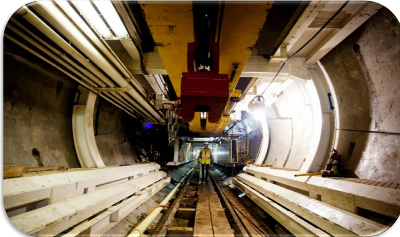
Nearly 1,000-ft of the five-mile-long Bay Tunnel have been completed, construction crews can still walk to the TBM. Later, cars that run on rail tracks will be lowered in to the tunnel to transport tools, material and workers when the tunnel extends further across the Bay.
