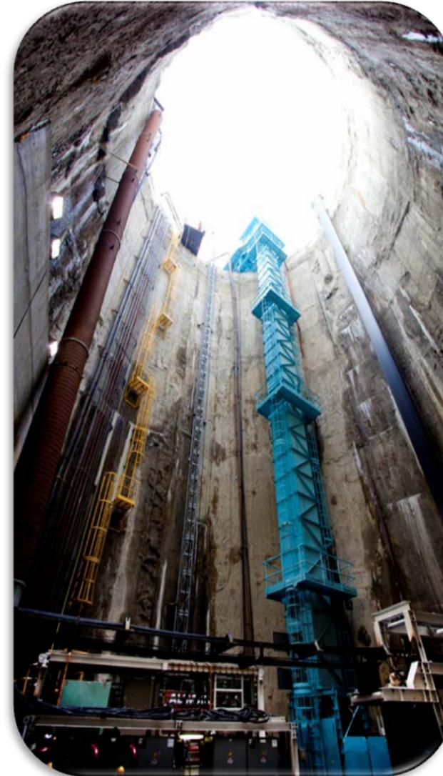
The Vertical Conveyor System in blue (above) lifts the spoils from inside the tunnel to the conveyor belt (below) and then transports the spoils to a nearby pit.
